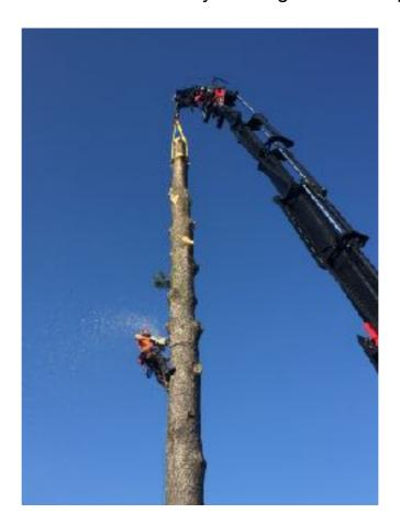
He added: "I am very impressed with the load cell. It is perfect for my application in weight, design, and ease of use. The data from the [load] cell allows me to pretension picks as the climber is cutting. As with any industrial lift evolution, weights, angles, and distances are essential
