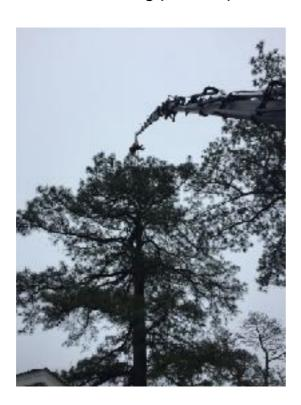
Wood weights were calculated in advance using a green weight log chart that provides a general guideline by species and size. On-site, the load cell recorded the smallest pick at 1,625 lbs. and the largest at 6,500 lbs.
